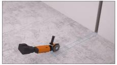
Before an installation carefully dry out and clean floor surface. Check fatness of the ground. Make a groove for a protective corrugated pipe.
