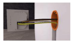
10. Connect the electric wires to the thermostat according to the thermostat instructions. Turn on system and verify its operation by infrared thermometer. inspect manually if it warms up. Low heating film power need few hours to warm up. Be patient.
