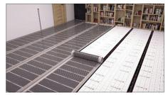
Distribute the heating film. Heating film will work both sides the same. Leave distance of approximately 50 mm from each wall, and at least 10 mm between strips.
