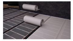
9. Lay down vapour barrier and secure with Termofol adhesive tape.
