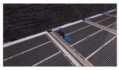
Using adhesive tape connect and secure heating film to insulation pads. Using appropriate tools attach clips to heating mat.
