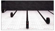
Place the insulation under the entire floor surface and secure with TERMOFOL tape. Spray glue is permitted.
