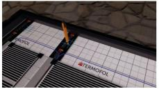
Secure all electrical connections with black, sticky butyl tape this include copper part on the other end. Secure electric wires and hearing film with Termofol adhesive tape.
