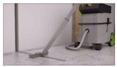
2. Clean the floor and install a protective NTC sensor pipe.
